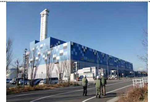
Power Station (LNG)
