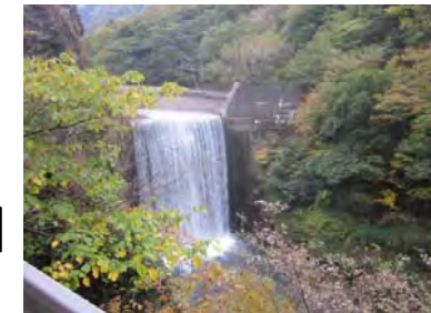
Hydro-electric power station with Erosion Control Dam
